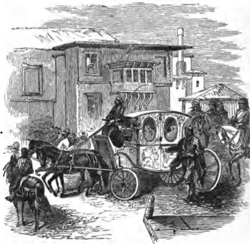
THE SULTAN GOING TO MOSQUE.
